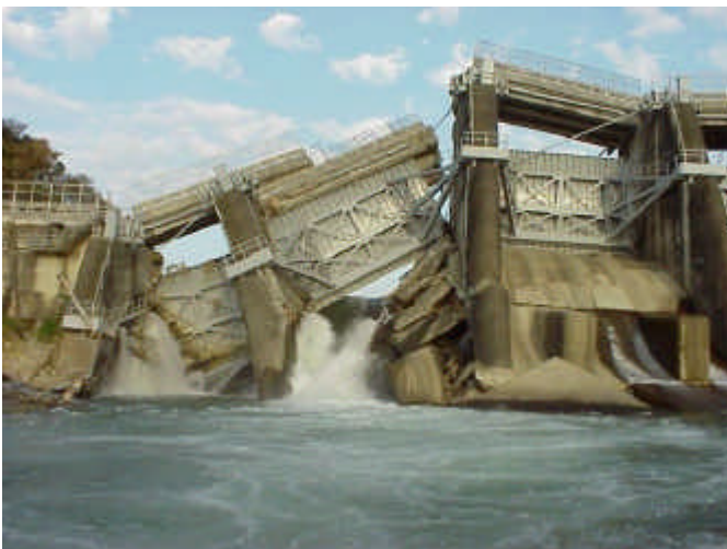
Fig. 2: Shih-Kang weir in Taiwan, destroyed by fault movement during the September 21, 1999 Chi-Chi earthquake
