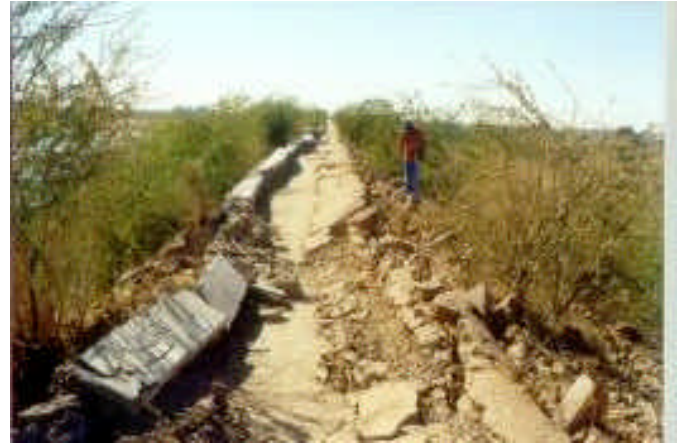
Fig. 3: Earth dam damaged by the January 26, 2001 Bhuj earthquake, Gujarat, India
