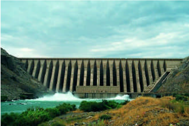
Fig.1: Sefid Rud buttress dam in Iran, damaged by the June 21, 1990 Manjil earthquake
