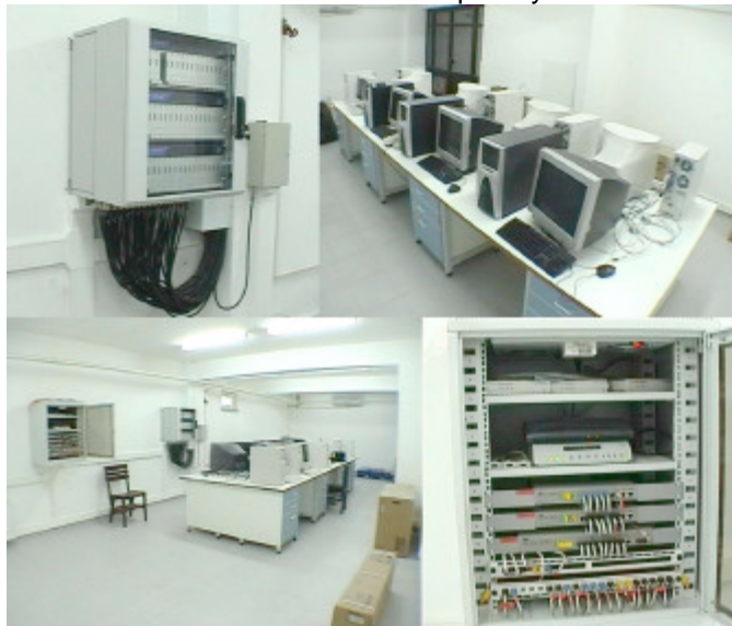
Figure 4. Main Data Center in KOERI during installation.
