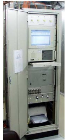
Figure 4. Seismic Safe CPU Cabinet in Beznau NPP.
