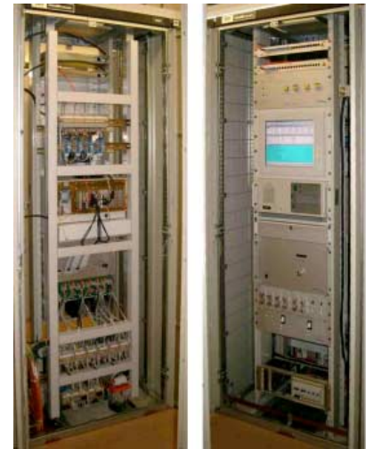
Figure 12. Reuse of the existing cabinet for the GeoSIG CPU in Leibstadt NPP.
