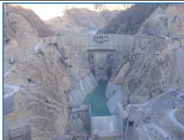
Figure 7. Karun III Dam and Plunge Pool.
