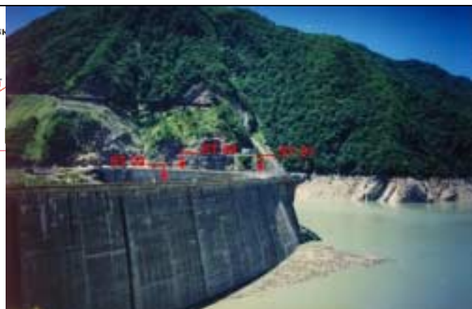
Figure 4. Location of the accelerometers on the crest of the dam
