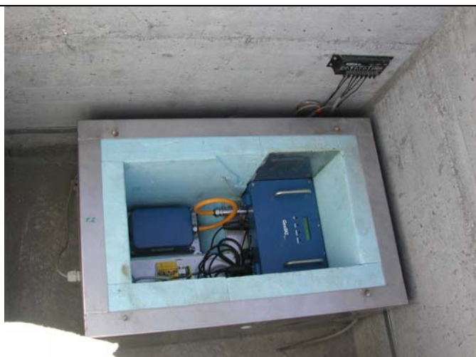
Figure 5. Strong Motion Station in Special Thermo-Insulated Housing
