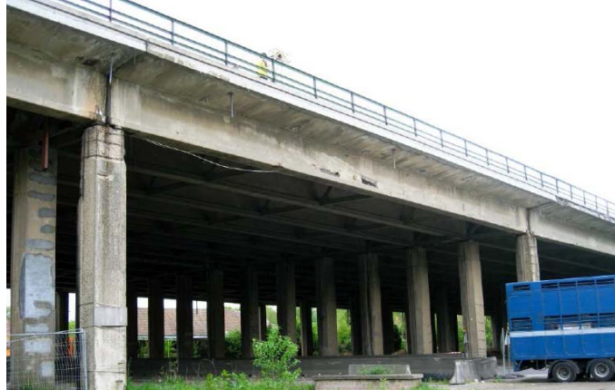
Figure 3. A south view of the Boirs viaduct, showing the severely damaged side girder of Span X.
