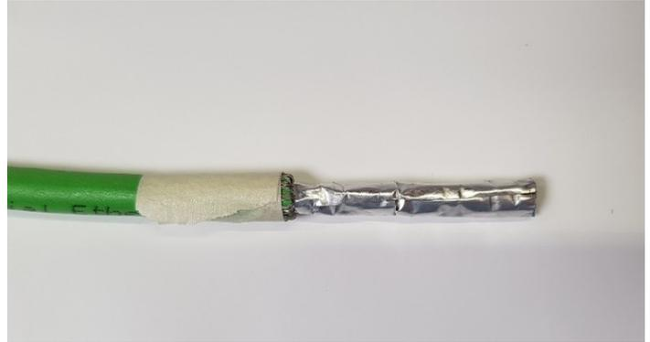
Figure 18. Apply tape on the shield
