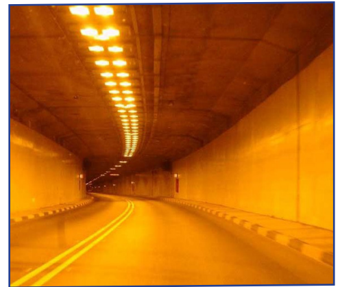
The undersea tunnel has a total road length of 910 meters and a maximum depth of 27 meters below sea level.
