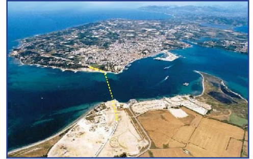
The Preveza-Aktio immersed tunnel crosses the strait that separates mainland Greece from Epirus in the Ambracian Gulf.
