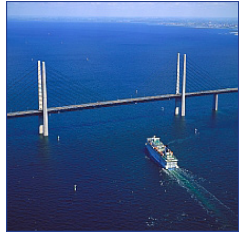
The Øresund Bridge is a combined railway and motorway cable-stayed bridge that is 7,845 m in length.
