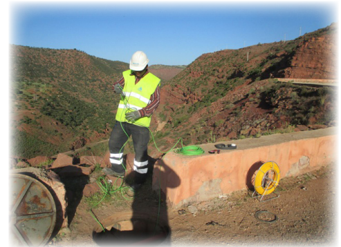
Installing digital cable for the seismic monitoring system.
