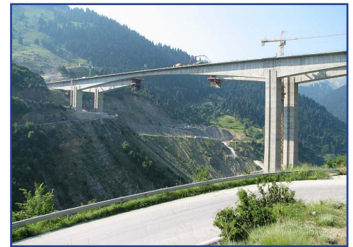
Metsovo Bridge is a single box girder bridge located in the north of Greece.
