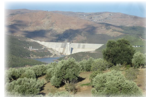
Wadi Martil Dam includes a concrete face fill dam on Wadi Mohjerat, and an earth fill secondary dam.
