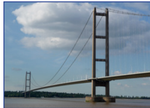
Humber Bridge required updating testing since previous efforts were analogue.
