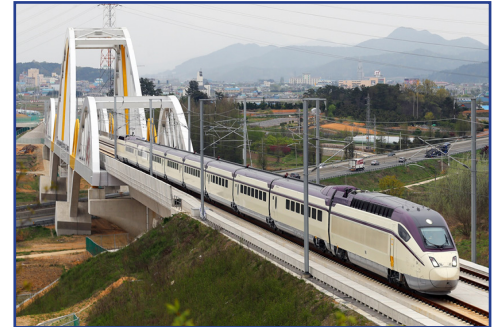
The Honam high-speed rail line for the new Korea Train Express.
