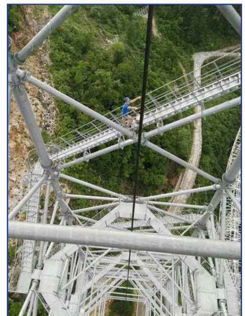
EPC engineer trekking to the top of a 150 m tower to install GMSplus.
