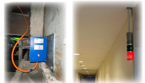
GeoSIG accelerometers (left) detect motion as part of the structural monitoring of the building. If the exceedance is deemed unsafe, red lights in the corridor (right) will alert people that evacuation is necessary.
