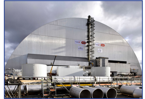
Construction of the new sarcophagus over the Chernobyl Unit 4 reactor.
