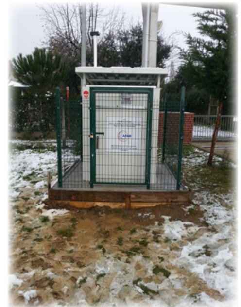
GeoSIG instruments are installed in seismic stations throughout Turkey as part of its strong motion network to continuously monitor seismic activity.
