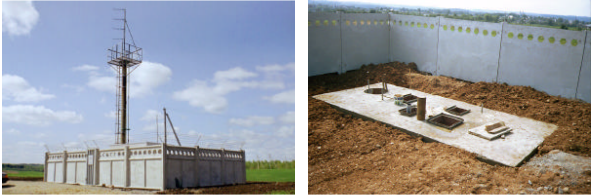
Fig. 3 Photograph of a typical seismic station (left: completed station with aerials for telemetry; right: foundation plate with openings for instrument locations)
